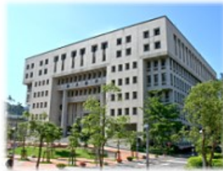
行政大樓 / Administration Building
